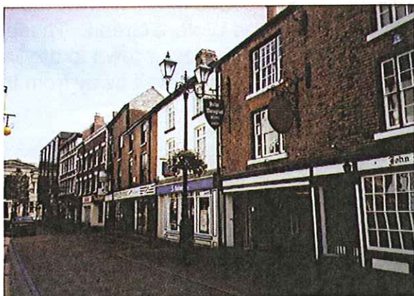
Entrance to Chestergate Mall, Chestergate
