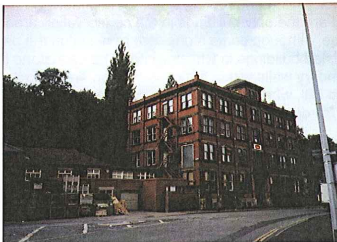
Former factory, Waters Green
