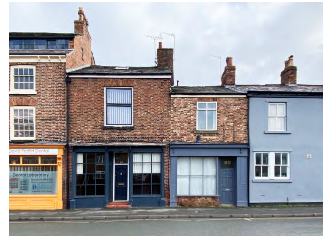
Shopfronts retained as part of change of use to maintain street frontage
