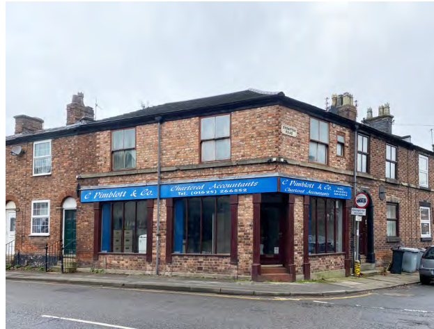
Shopfront and entrance addressing street corner
