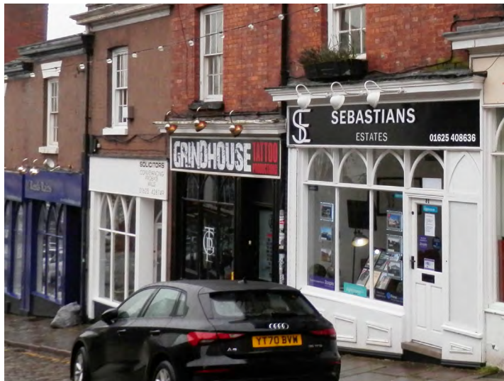
Lighting and pointed arch detail to transom lights
