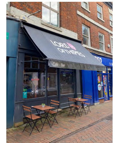
Retracting awning with metal arms
