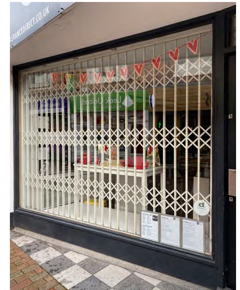
Internal lattice shutter
