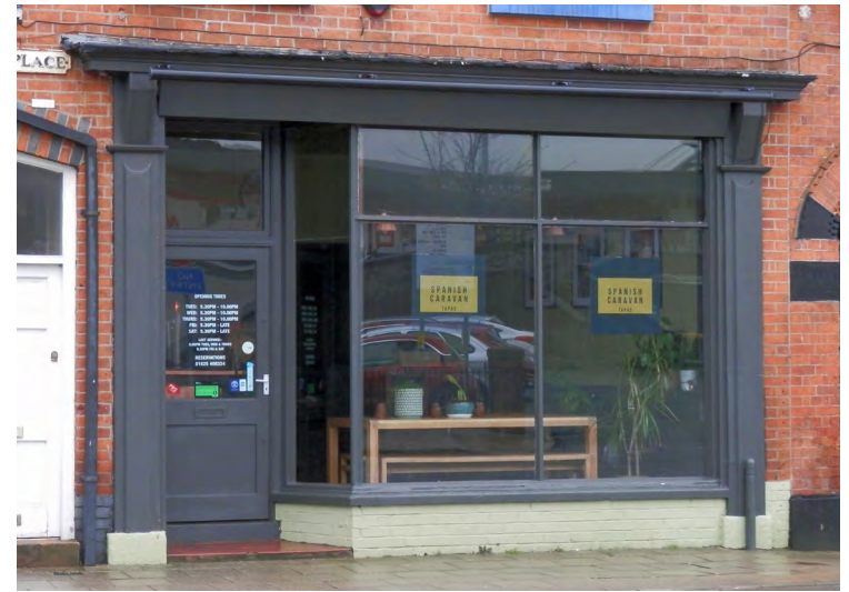
Appropriately detailed replacement shopfront retaining pilasters
