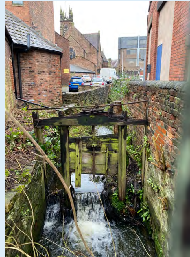
Pickford Street sluice
