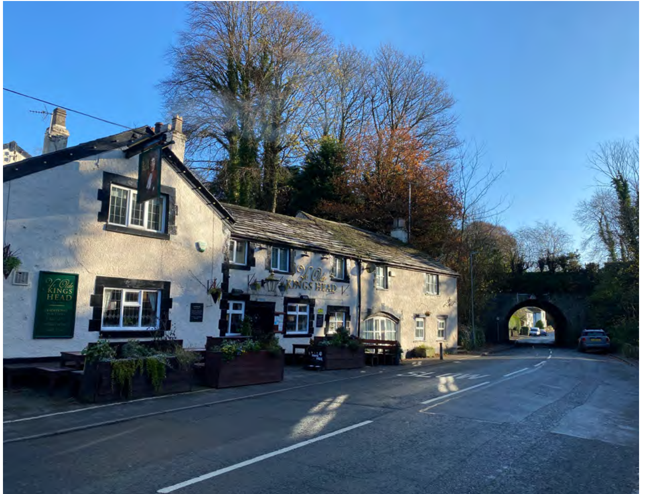
E.4 Ye Old Kings Head and Gurnett Aquaduct
