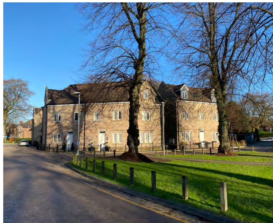
West Park Mews development around the historic Macclesfield General Hospital blocks
