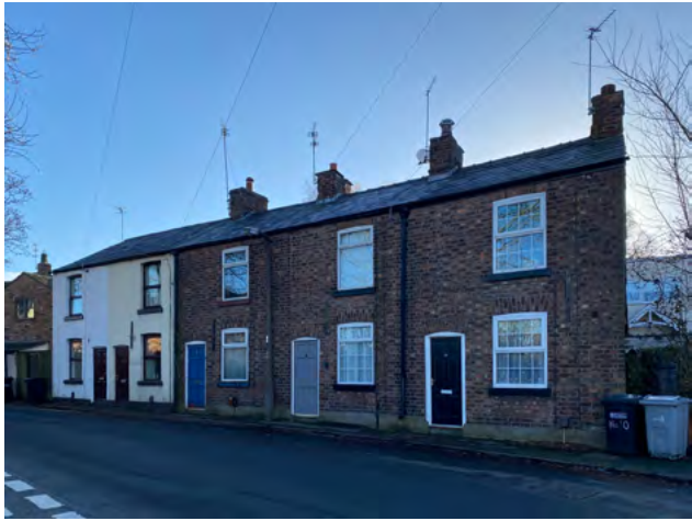
G.5 19 th century workers cottages on Chelford Road
