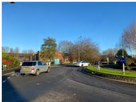
G.2 Cumberland Street cutting through area
