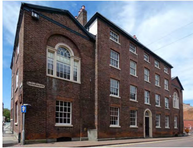
A.4 19 King Edward House, Jordangate
