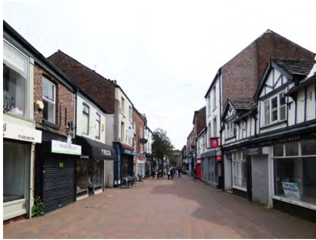
A.5 View east along Chestergate
