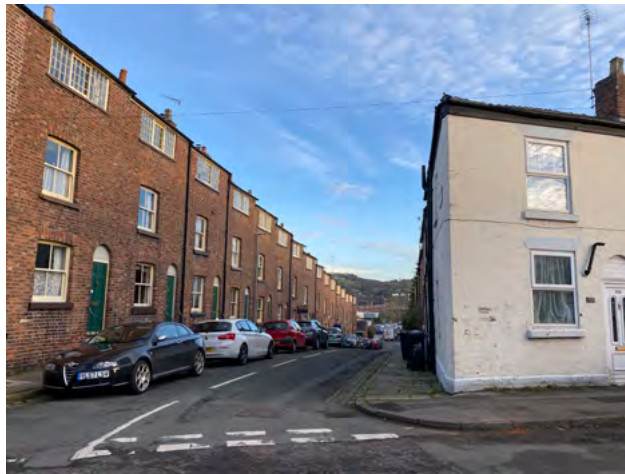
B.5 View east along Paradise Street
