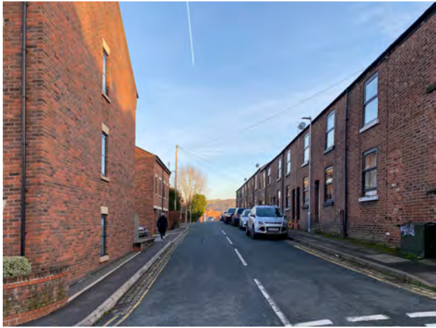
B.5 View east along Parr Street
