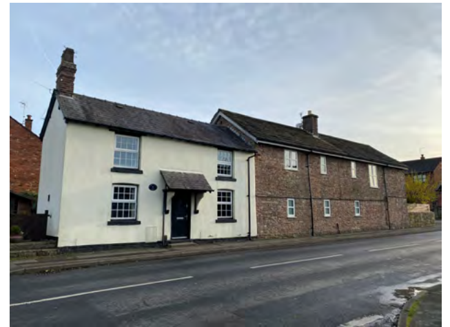
F.2 Pump Tree Farm, Broken Cross
