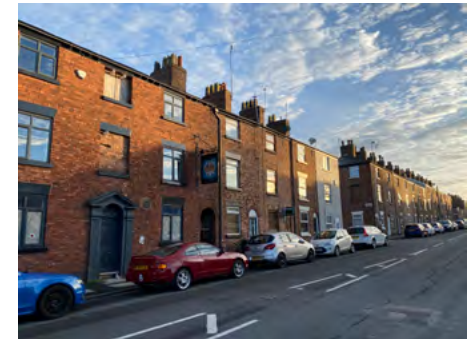
B.2 North end of Bond Street
