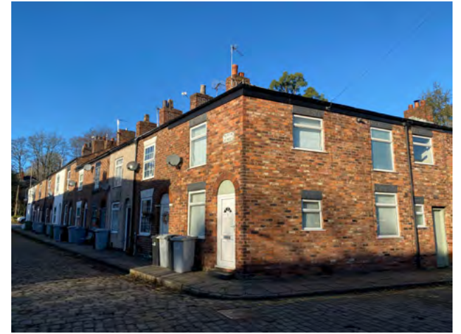
G.2 Pocket of workers cottages on Nixon Street
