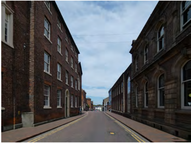
A.5 View north along Jordangate
