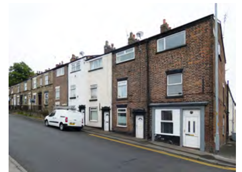
C.2 Former mill weavers cottages
