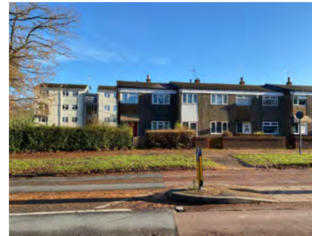
G.2 Housing estate on Priory Lane
