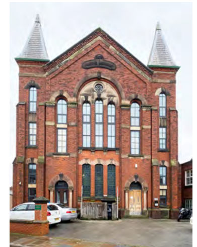
Converted Primitive Methodist Church with contemporary windows suited to architectural style
