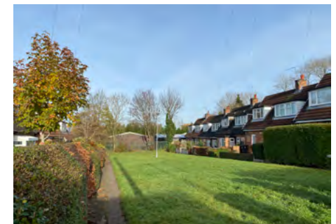
F.2 Green frontages in place of roads and parking in Weston Estate
