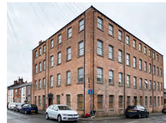
The Silk Factory converted to domestic use with appropriate alterations
