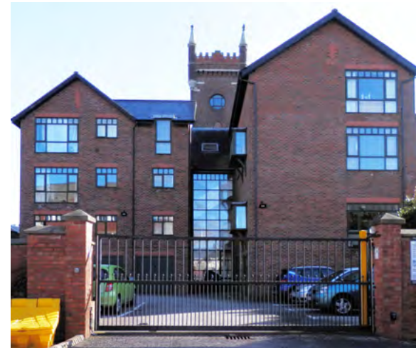
The Tower House contextual rear extensions
