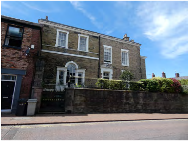
A.4 Cumberland House, 9 Jordangate
