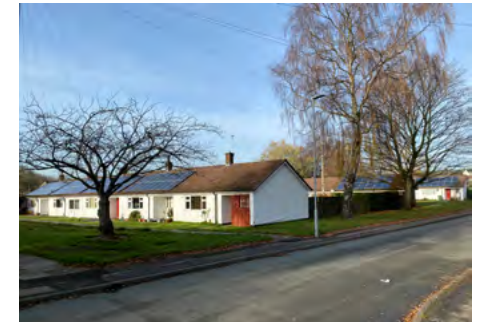
F.2 Bungalows set around green spaces within Weston Estate
