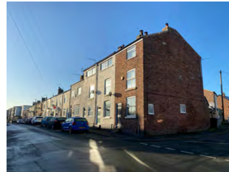
E.2 Three storey weavers garrets and two storey mill workers cottages
