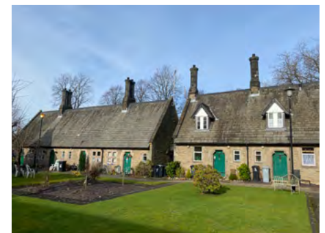
B.2 Stanley and Brocklehurst Almshouses
