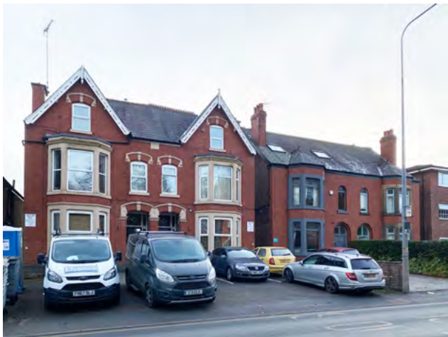
F.2 Victorian villas on Chester Road
