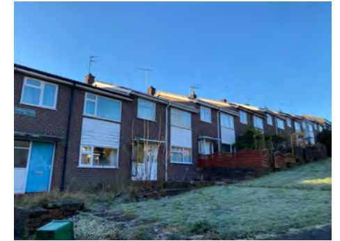
H.2 Bollinbrook Estate terrace
