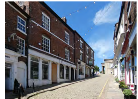
A.2 Church Street leading to Market Place
