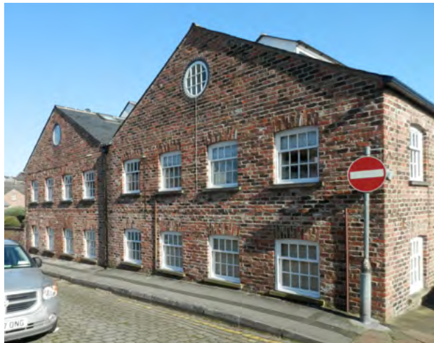
Regent's Foundry sensitive residential conversion
