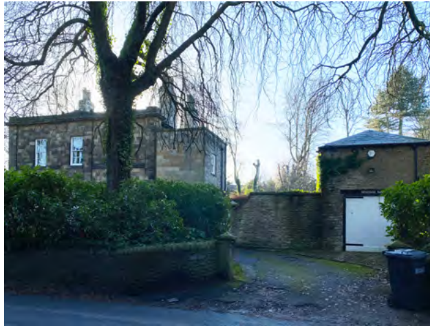
G.4 Macclesfield District General Hospital (original blocks)
