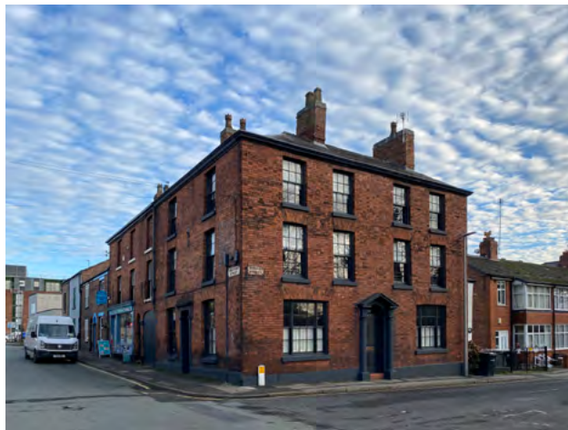
B.4 36 Bridge Street, 26, 28 and 30 Great King Street
