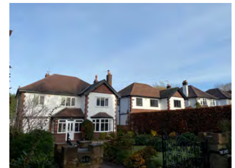
F.2 Interwar housing on Ivy Lane
