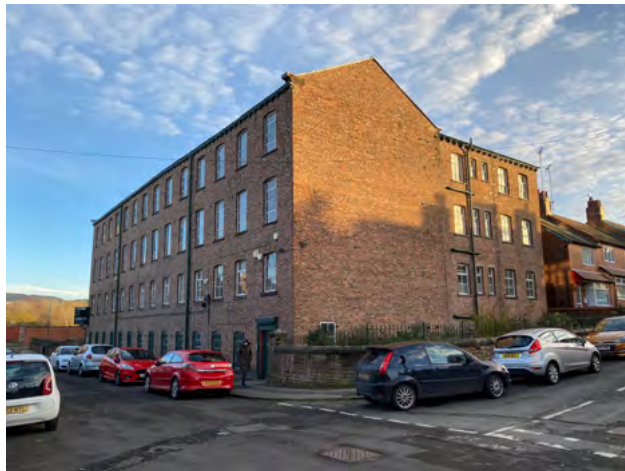
B.4 Newbridge House, Henderson Street
