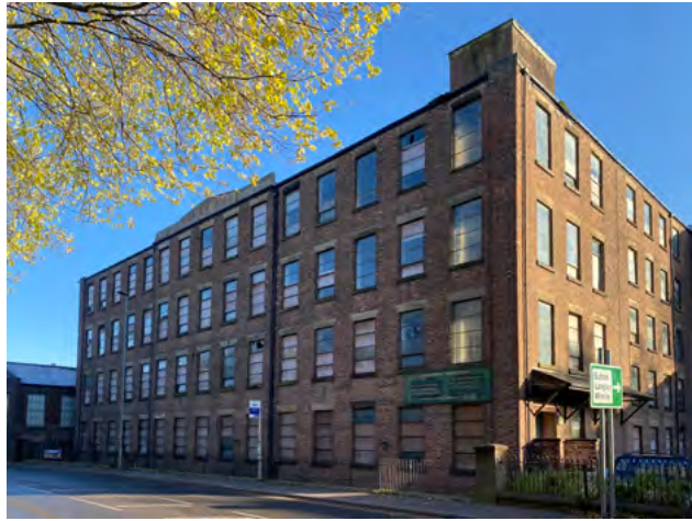
E.4 Albion Mill, London Road
