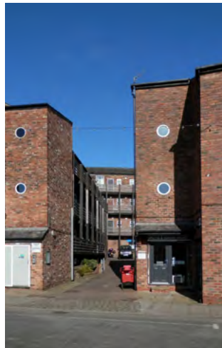
Sensitive contemporary alteration to Royal George Mill to form George's Court
