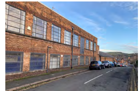
B.2 Bridge Street and Brookside Mills
