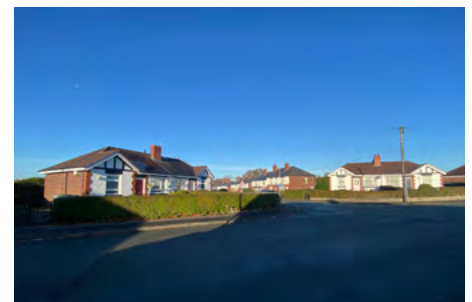
E.2 Decorative interwar bungalows southeast of South Park
