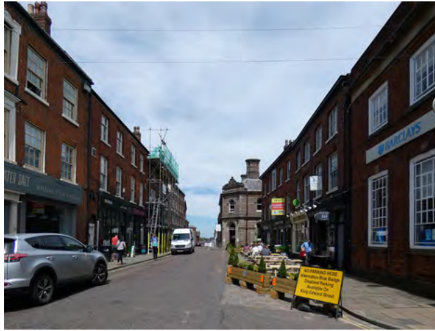
A.5 View north along Market Place
