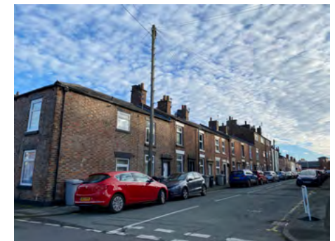
B.2 Mill workers cottages and weavers garrets on Brock Street
