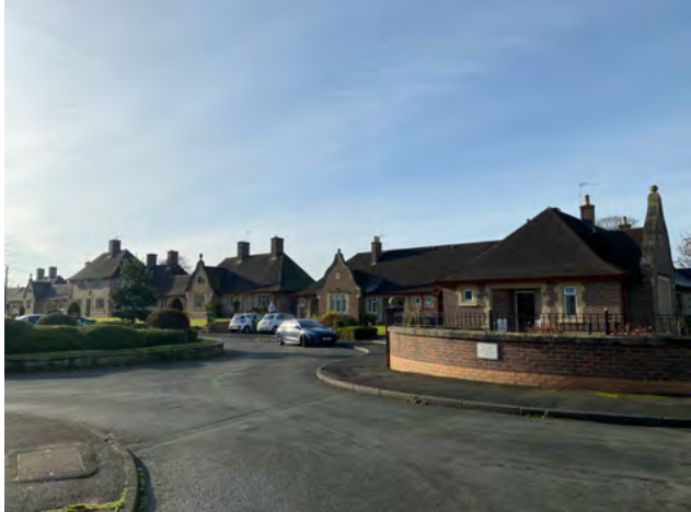
E.4 The Harry Turner Almshouses
